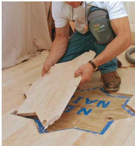
**Cutting corners.** A corner chisel squares off rounded corners left by the router bit.
