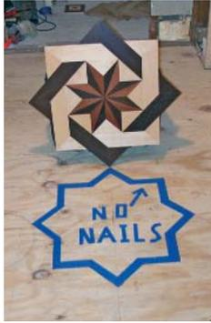
**A safe rout.** It's smart to mark the medallion's location before you begin to install the flooring. It's an easy way to avoid driving nails where they might make contact with the router bit.
