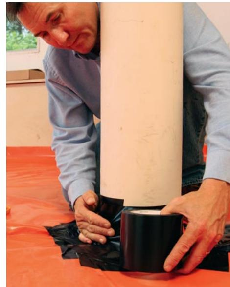
**Detail penetrations with a boot.** Cut the vapor retarder to fit around the base of the support as closely as possible. Although you can tape the penetration, it's better to create a boot out of excess material with splayed tabs. Tape each tab to the vapor retarder, then seal off all edges with the tape. The tape and the vapor retarder secured to the post can be trimmed with a utility knife to the proper height once the subfloor and flooring are installed.
