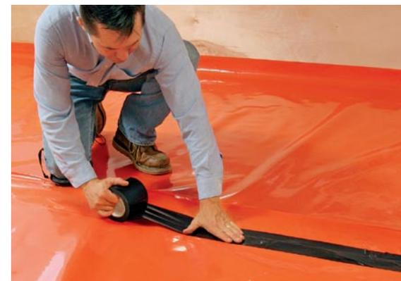
**Overlap and tape the seams.** The vapor retarder should extend to a point just below the top of the baseboard on the wall. Seams should be lapped by 1 ft. and be sealed with waterproof tape.
